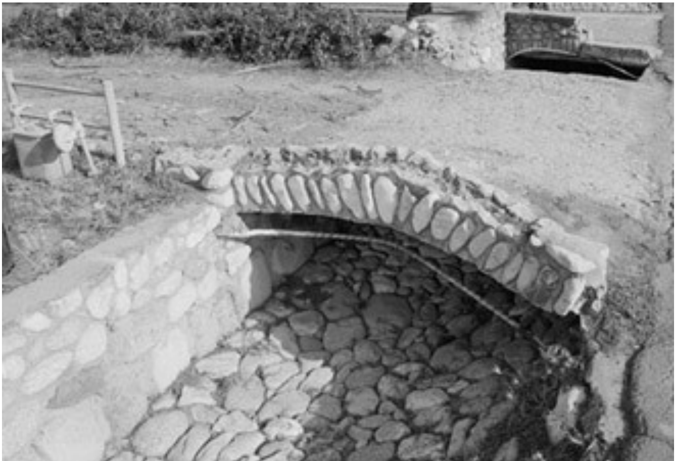
Example of rock curb with channel for water runoff
